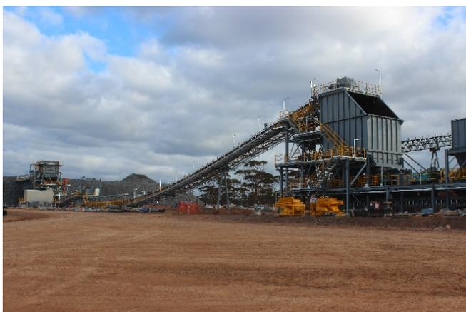
*Figure 5: Crushing Circuit*
