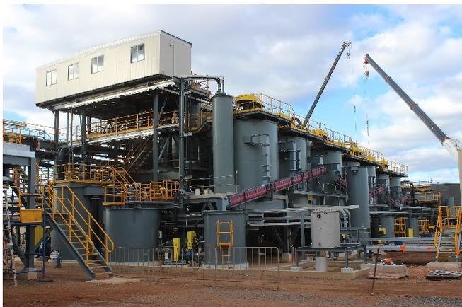
*Figure 7: Flotation Circuit (Copper side)*
