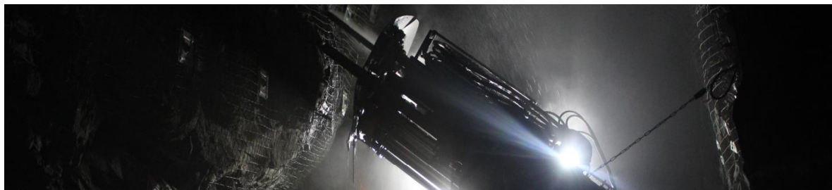
Stope production drilling in Nova underground
