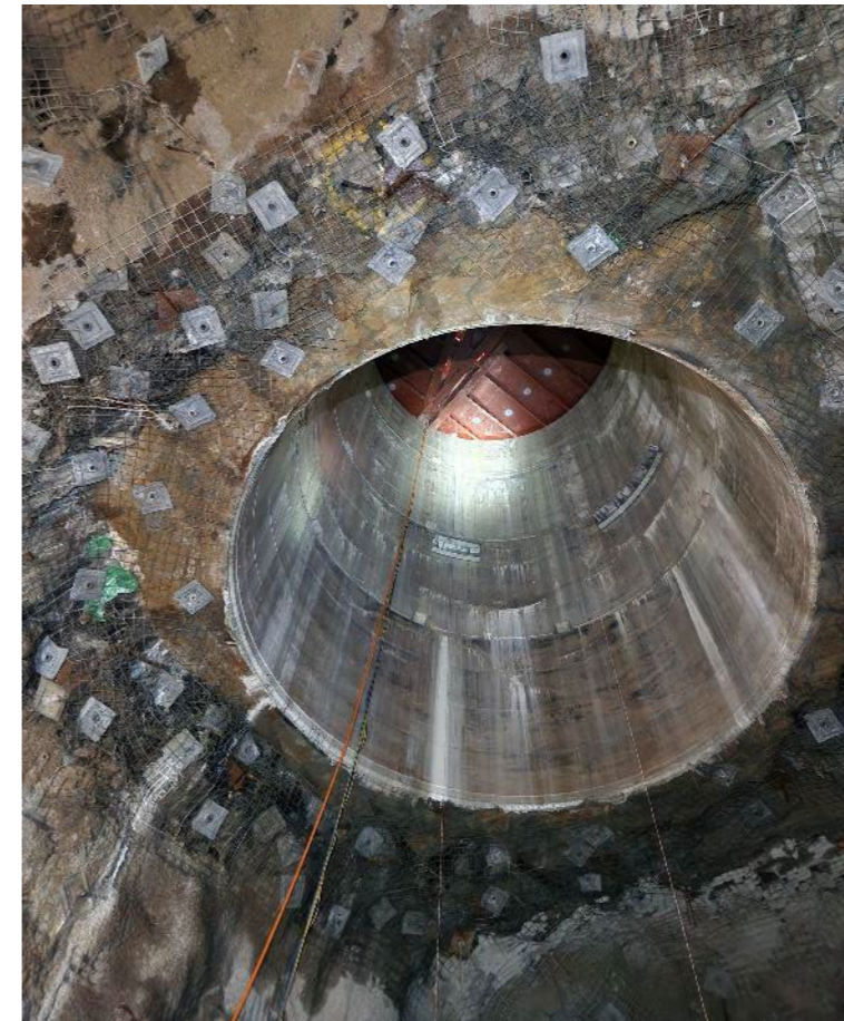
Current lined shaft, image from ground up
