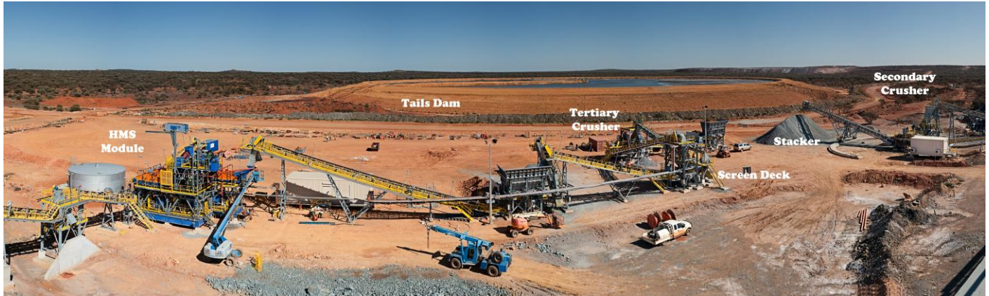
Photo 1: Jaguar HMS Plant Commissioning
