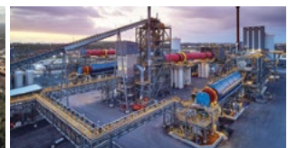
Kwinana Refinery Lithium hydroxide IGO 49%
