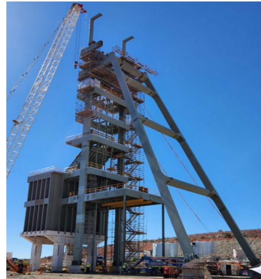
Cosmos headframe nearing completion
