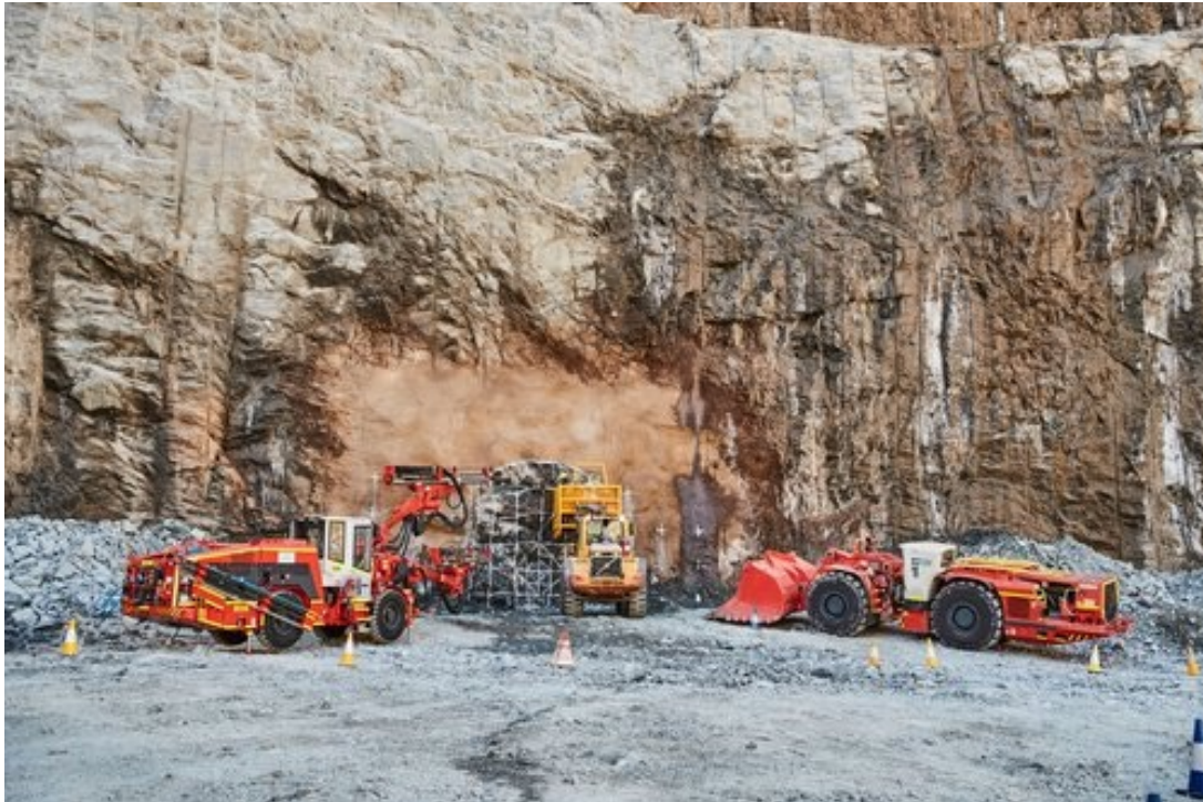
First blast for the portal at Boston Shaker on 8 May 2019
