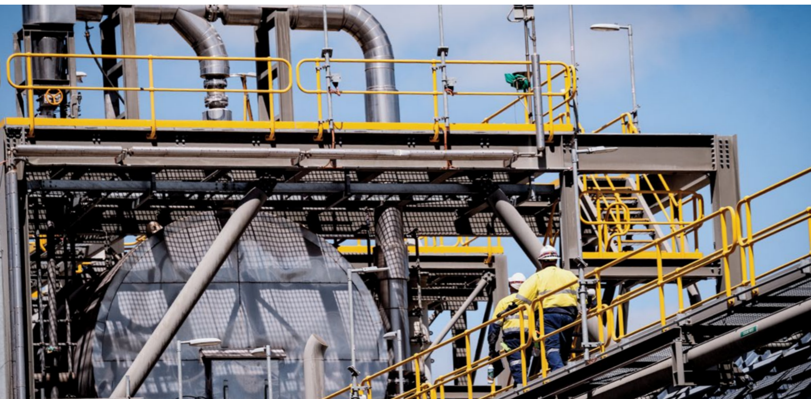
Kwinana Lithium Hydroxide Refinery
